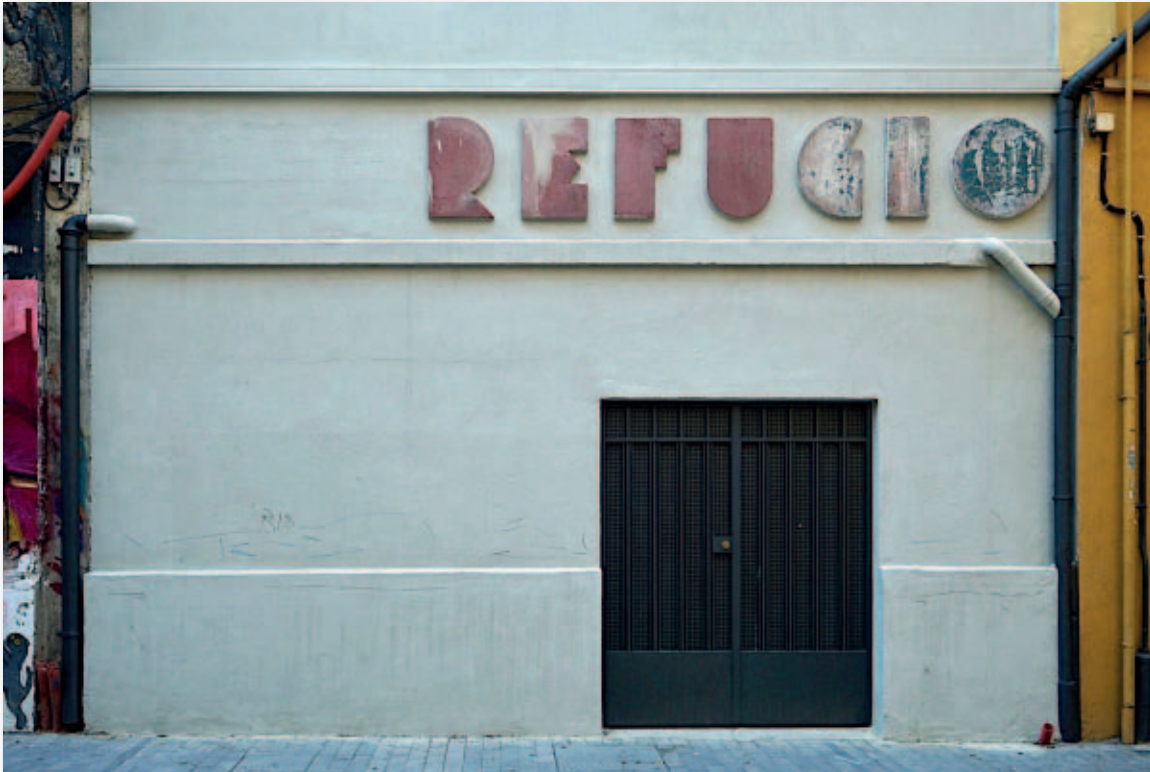
Façade of the air-raid shelter at the intersection of Carrer (street) dels Serrans and Carrer de Palomino with its characteristic Art Deco lettering, taken during its restoration process. Photo by José M a Azkárraga (Valencia, May 2017).
